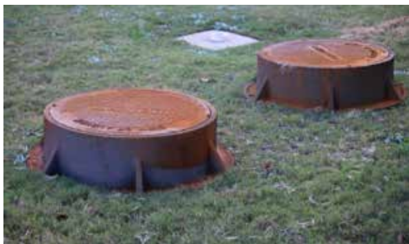
Cast iron cover securing grease trap.
